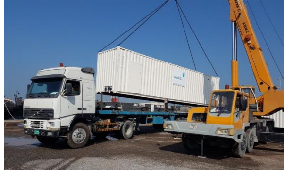
Loading emergency desalination plant onto ship for journey to Cape Town
